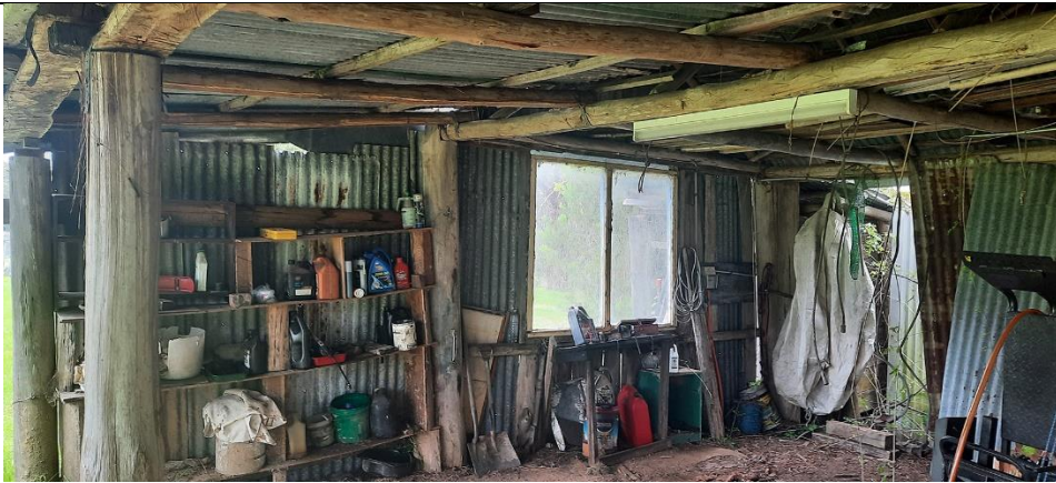
Shed interior showing pole framing.
